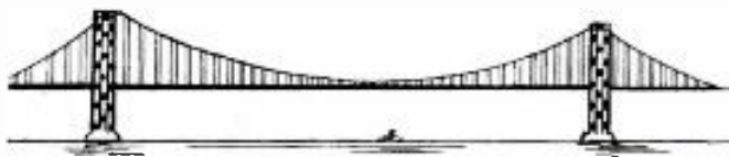
George Washington Bridge
